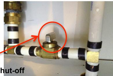
CLOSED POSITION: Shut-off valve handle in opposite direction of pipe.
