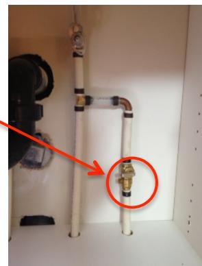
CLOSED POSITION: Shut-off valve handle in opposite direction of pipe.
