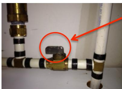
OPEN POSITION: Shut-off valve handle in same direction as pipe.
